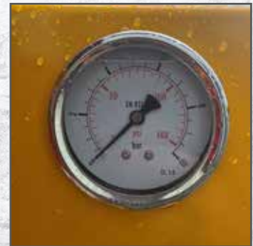
Manometer for checking liquid
